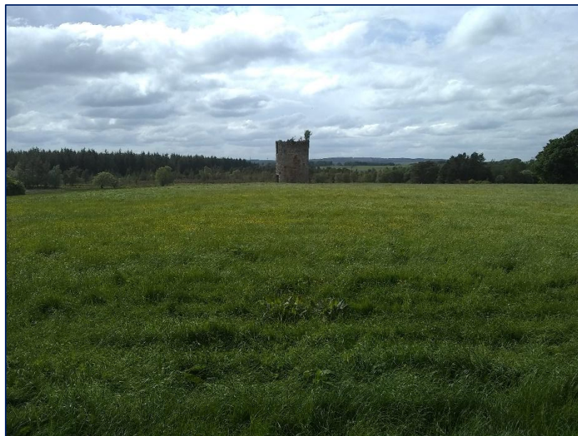
Plate 28: West facing view of the Category C Listed Pigeon Tower at Lawhead (Asset 10)
