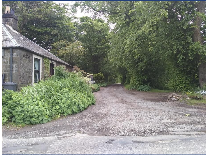
Plate 37: South facing view towards the Category B Listed Auchenhard House (Asset 24) and Auchenhard Farmhouse (Asset 25)
