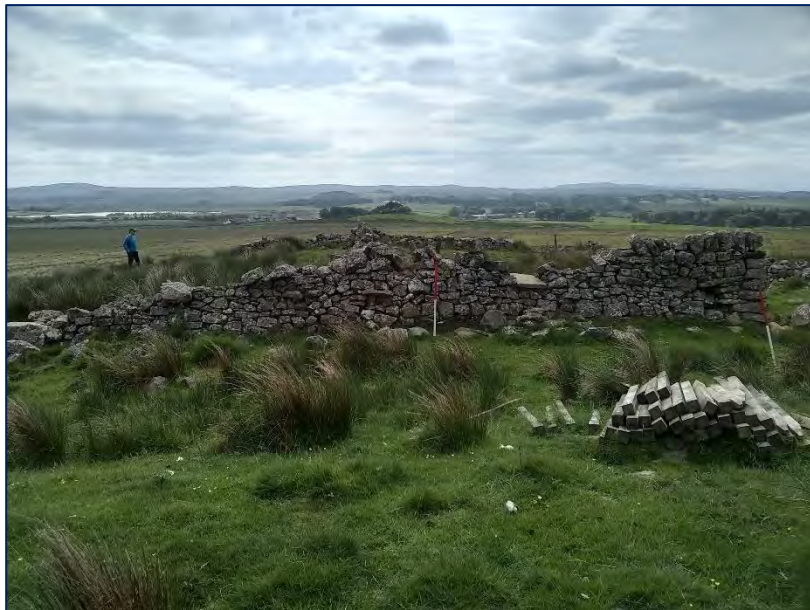
Plate 7: South facing view of the building remains at Site 88
